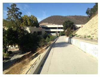
Photo-3 Paved walkway from main campus to student parking lot does not appear to meet accessibility requirements.
