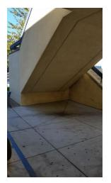
Photo -1 Lack of physical barrier below stairs.
